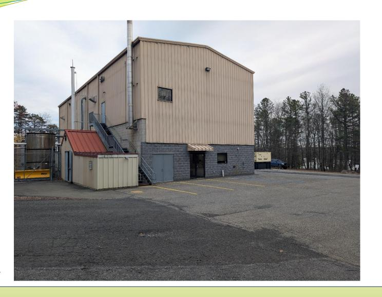
This is the entrance to the production facility. The production facility is 40 feet high and 42 feet wide. A generator can be seen to the right of the building that can power the entire plant from the most basic 120 volt outlet to the 480 volt motors operating in the plant.
